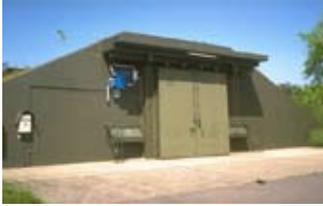
Ammunition is typically stored in magazines which are partly earth covered. Usually, ammunition magazines have a high humidity inside, resulting in corrosion damage and the quick decomposition of chemical compounds. Munters sorption dehumidifiers create an environment where corrosion is slowed down and the safe life of the ammunition is extended.
